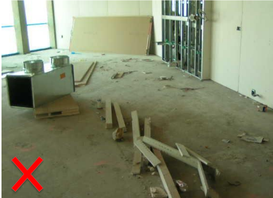
Interior housekeeping is poor in this example – workers lifting and moving materials would be exposed to potential trip and fall hazards.
